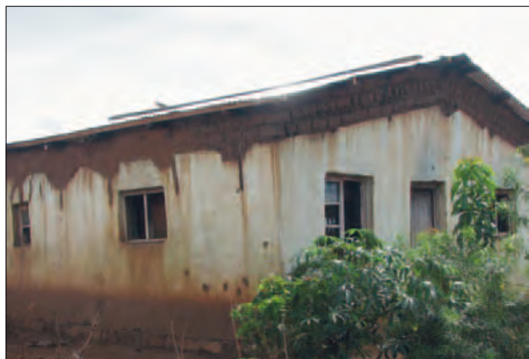
Figure 16. Roof failures in CCODE housing Area 49, Lilongwe have led to emergency repair and rebedding of roof tiles
